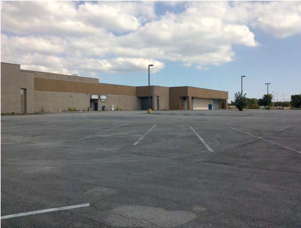
Photo 01 View of BX building and parking lot on eastern portion of site
